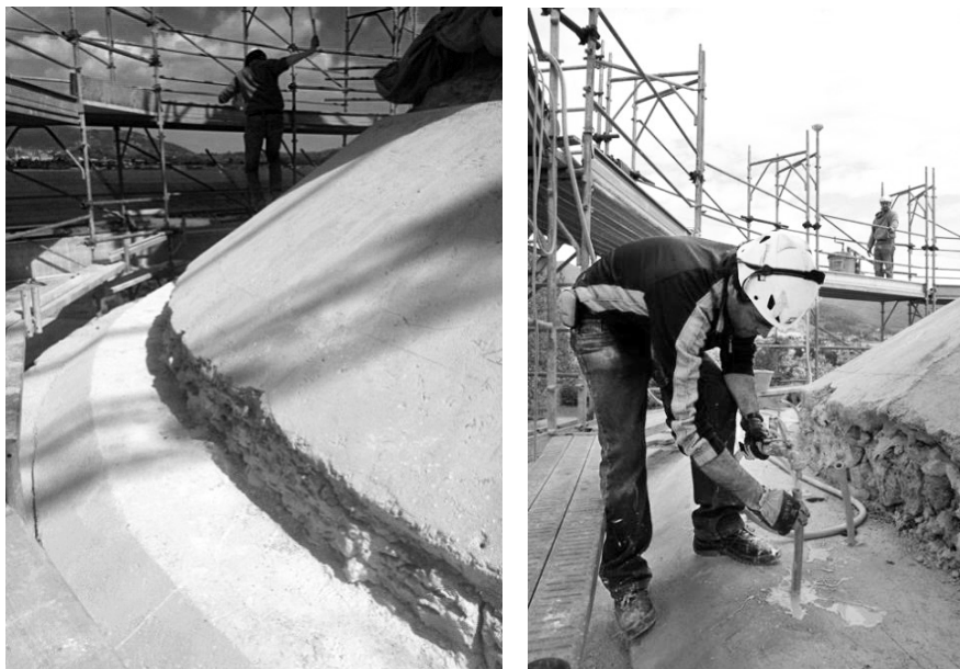
Figure 11. Preparation of the vault for the installation of the lower ring and consolidation of the upper layer of the perimetral masonry by grouting with lime mortar
