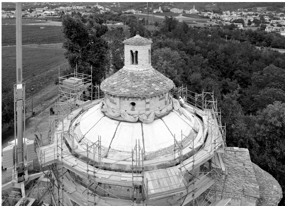
Figure 14. General view of the complete installation of the steel strengthening system
