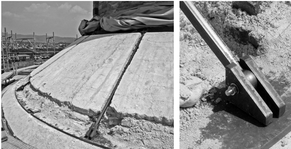
Figure 13. Connection between the upper ring to the lower and detail of the connection of the tendon to the lower ring.
