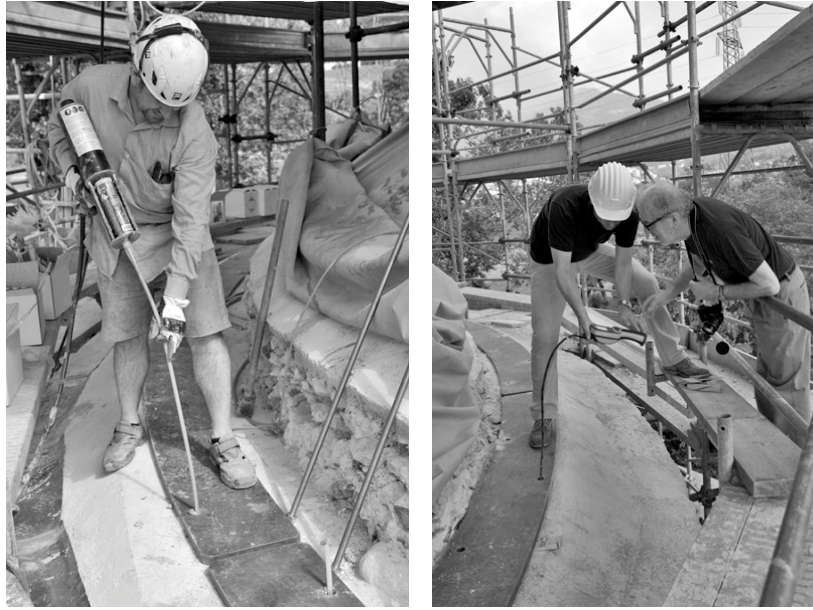
Figure 12. Grouting with lime mortar of the steel anchors which connect the steel ring to the masonry and investigation of the boreholes with video-camera
