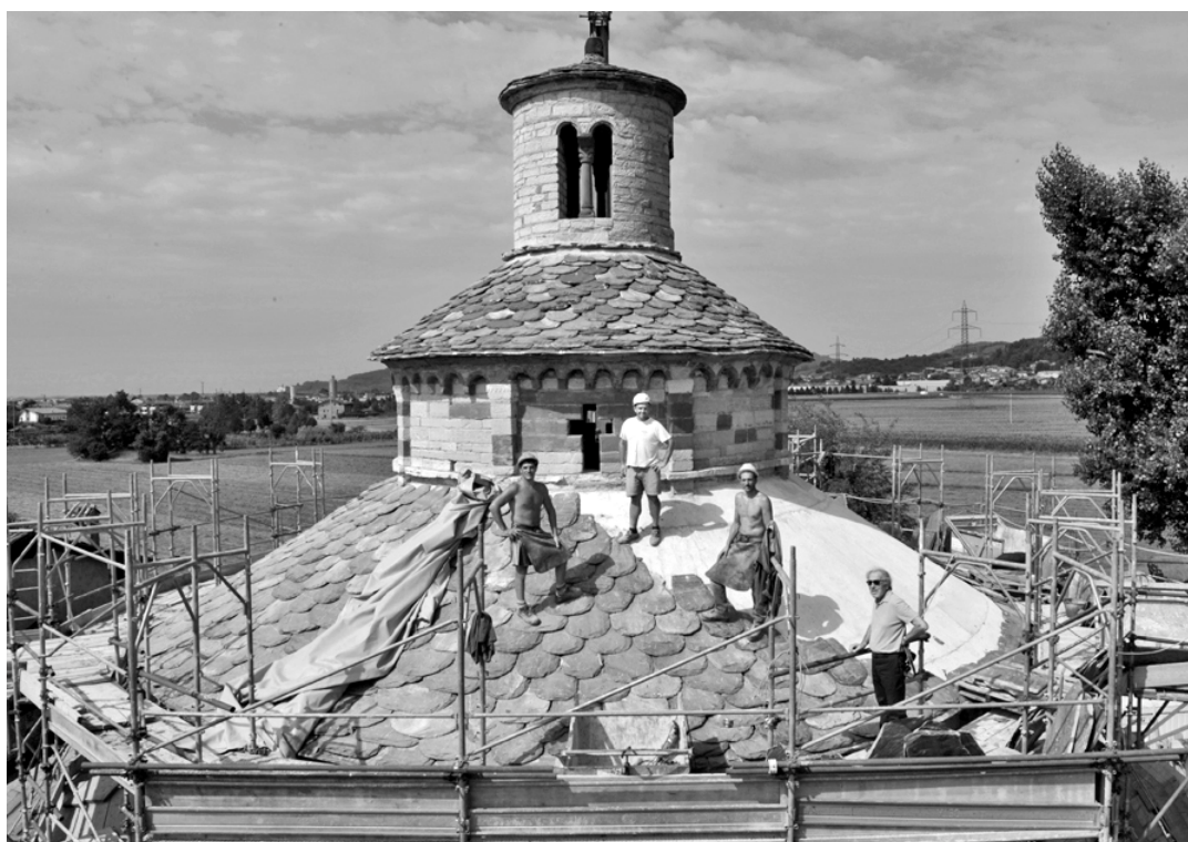
Figure 15. Final step of the straightening intervention: the placing of the stone slabs on the roof.
