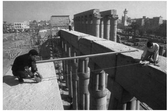
Fig. 4 – Measurements of relative displacements (manual system). Long base removable mechanical extensometer for measuring of relative displacements between the columns of Luxor Temple (Egypt), during the restoration phases.
