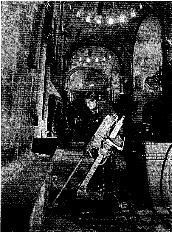
Fig. 3 - Drilling equipment for coring the foundation masonry
